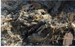
After being flushed, maintenance workers will often find baby wipes after they have gone through the collection system. They will get stuck in pump stations. The baby wipe below was found in a pump station causing the need for debris to be removed manually.
